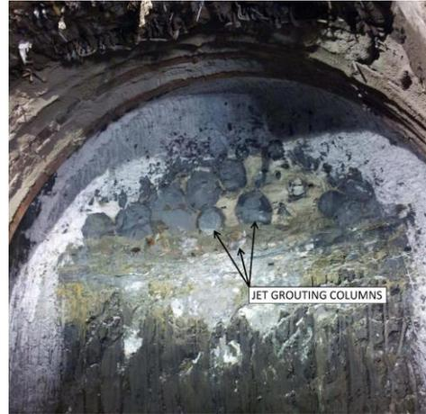
Figure 11. Face of the South East tunnel at 4th rib.
