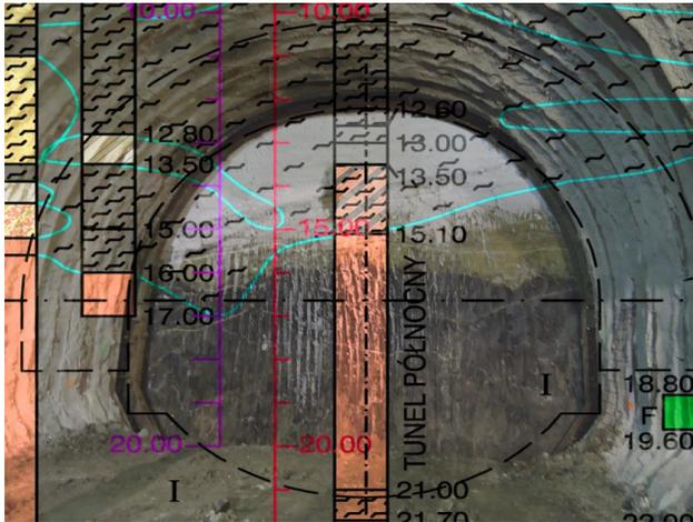
Figure 10. The design stratigraphy overlaying the North East face tunnel at 12th rib.
