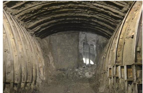
Figure 13. Central tunnel in the proximity of the last barrette to be demolished. On the right side the deactivated freezing pipes.
